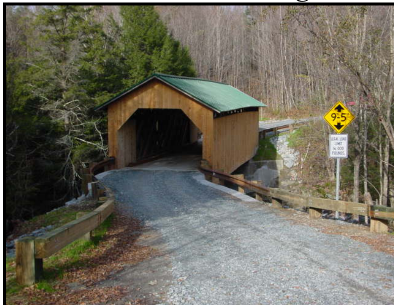
Creamery Bridge Both Restored in 2010
